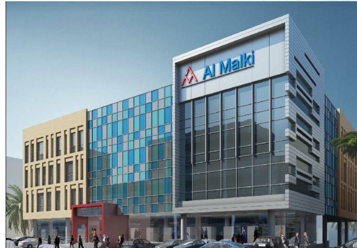
Located on the 2nd Floor of the Al Malki HQ Building on New Al Mirqab, Jawaan Street in Doha
